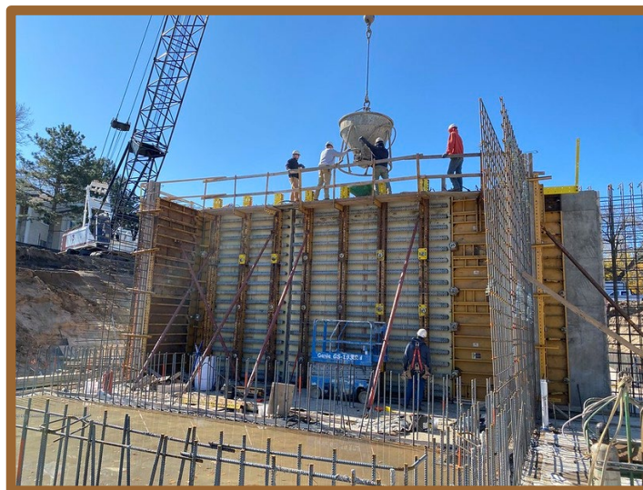
City of Robbinsdale Construction of a New Drinking Water Treatment Plant
